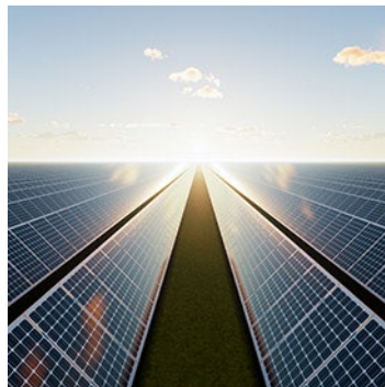
1500 V utility scale solar and BESS
