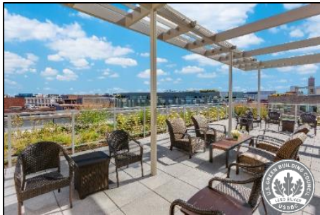
Green roof at Hilton Garden Inn M Street, Washington, DC, a LEED Silver hotel
