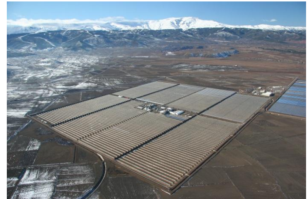
* Solana Project, Arizona
