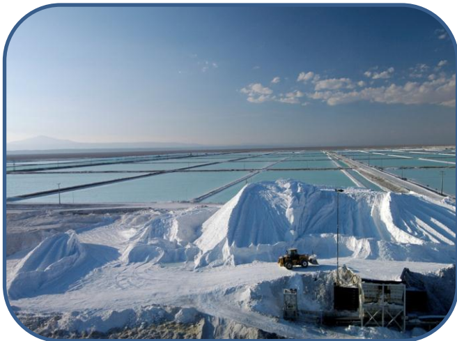
Photo: Evaporation ponds and silvinites stock pile, Salar de Atacama
