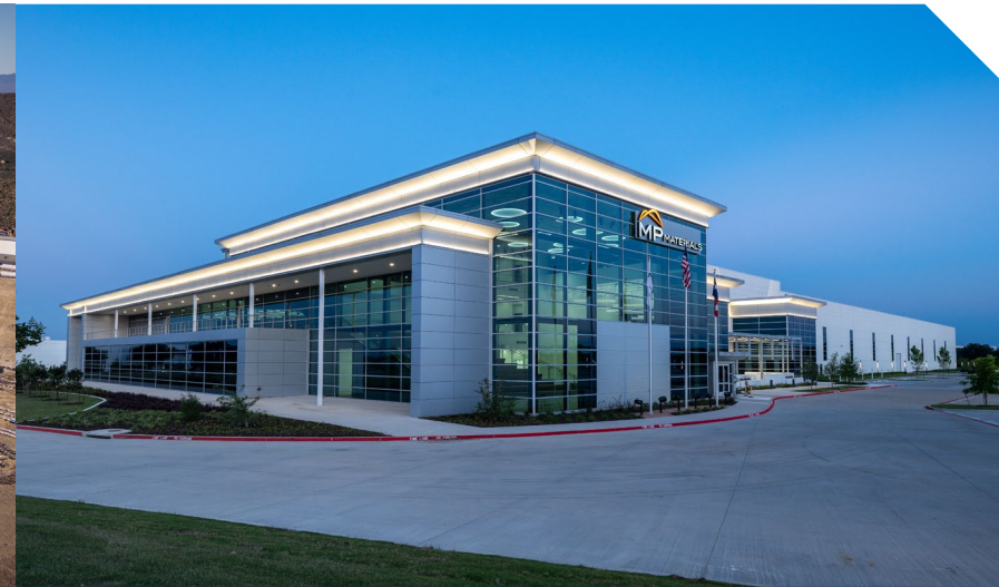
Downstream Metal, Alloy & Magnet Manufacturing
