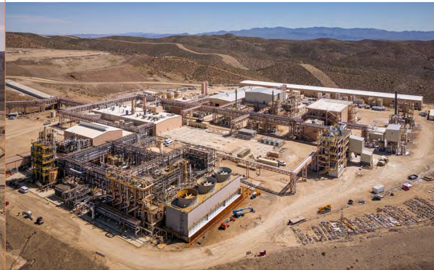
Midstream Separation & Refining
