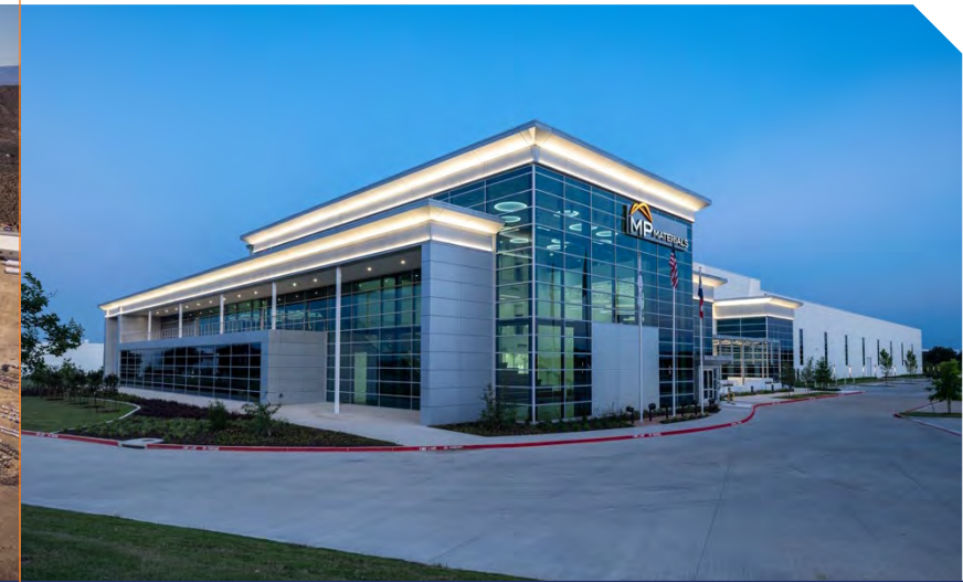
Downstream Metal, Alloy & Magnet Manufacturing
