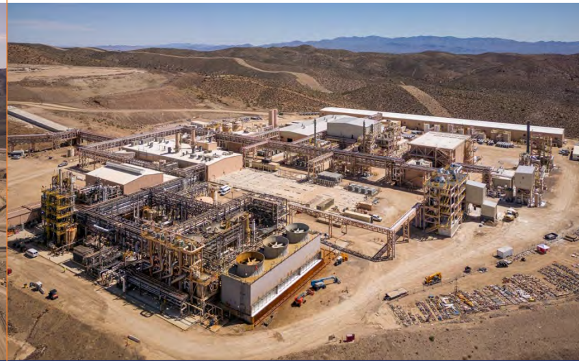
Midstream Separation & Refining
