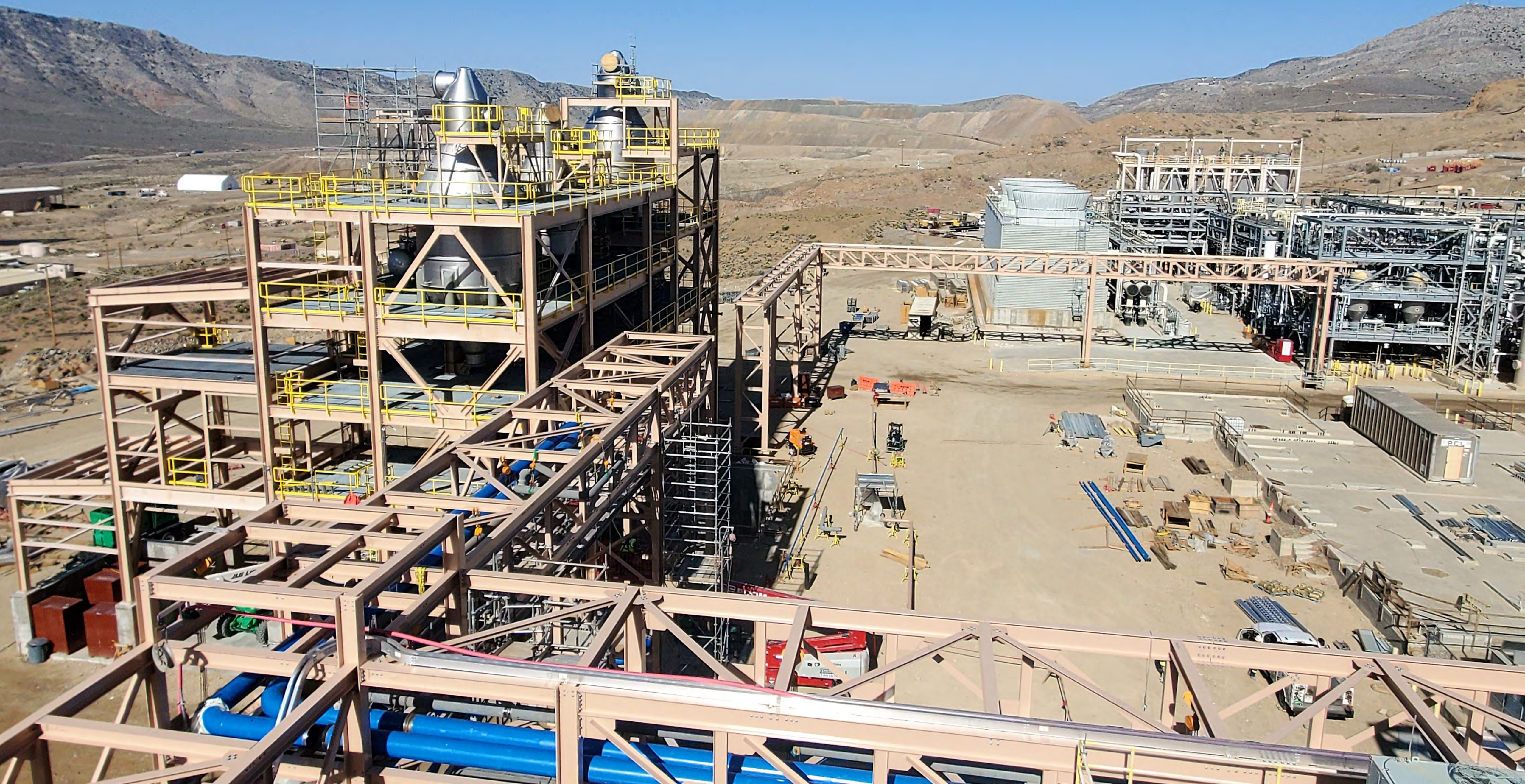
Salt crystallizer and brine concentrator
