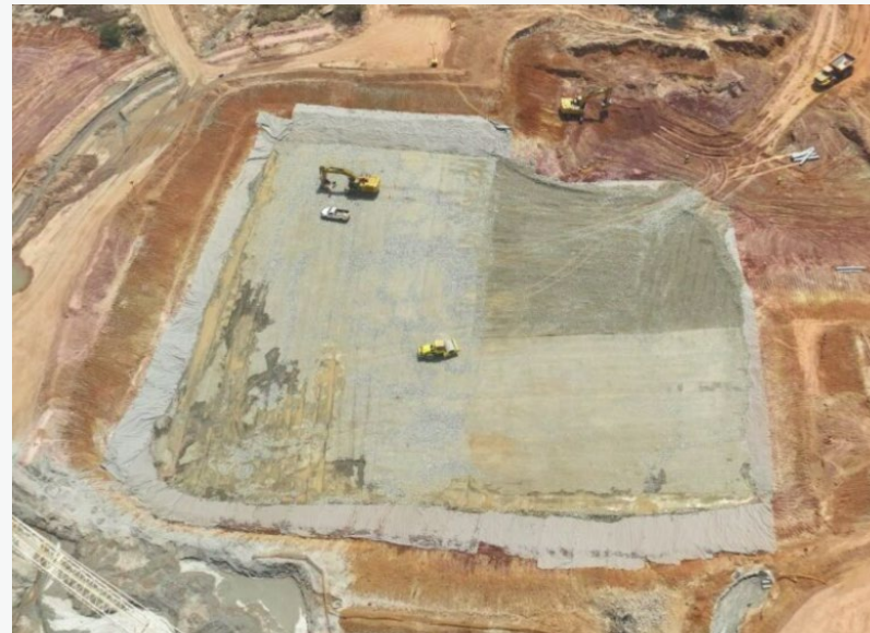
Mill Building Foundation
