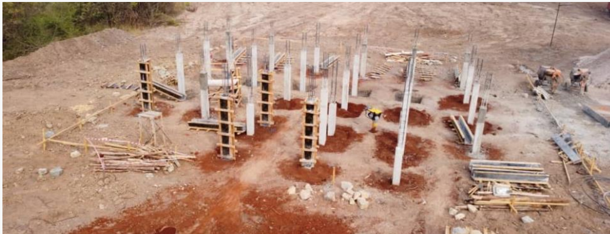
Mixing chamber and flocculator construction
