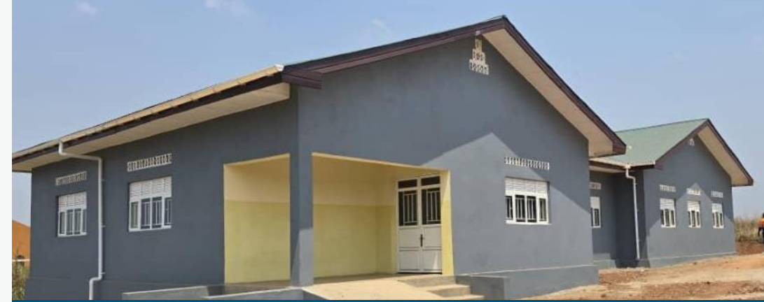
Construction of new maternity wing at Avokala Hospital
