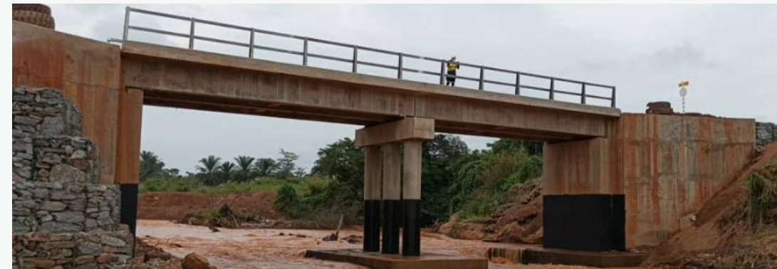
Completion of Lowa Bridge
