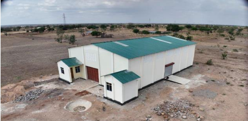
500Mt warehouse and processing facility
