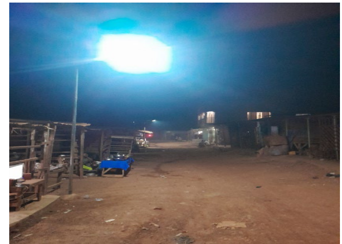
Solar Lamps installed in DK
