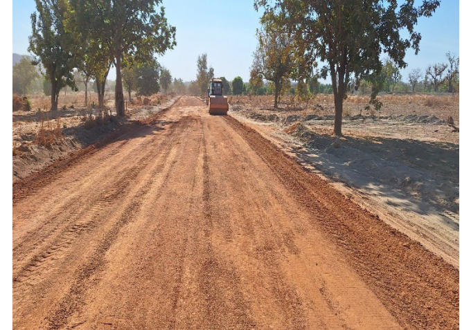
Dabara-Sakola road rehabilitation
