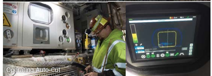
Road Header Cutting South Zone
