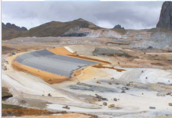
Process plant foundation Heap Leach Construction
