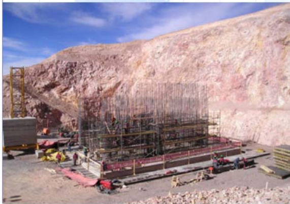
Construction of the valley-fill heap leach Foundation of the primary crusher
