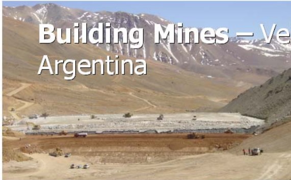
Construction of the valley-fill heap leach Foundation of the primary crusher
