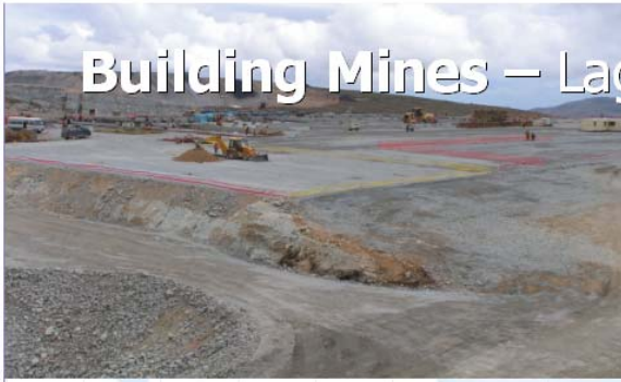
Process plant foundation Heap Leach Construction
