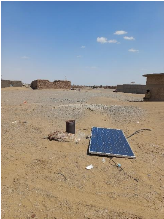
Borehole at W54 – Rajai
