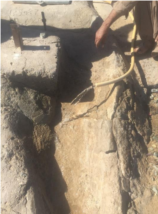
Dug well at W16 – Nok Chah
