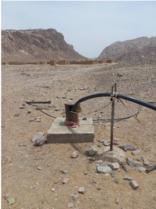
Borehole at W1 – Humai
