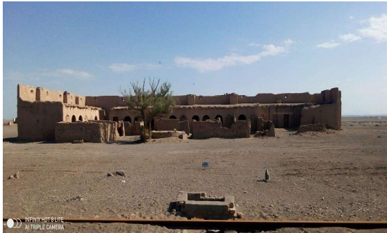
General view of the Koh-i-Daleel Railway Station from the south
