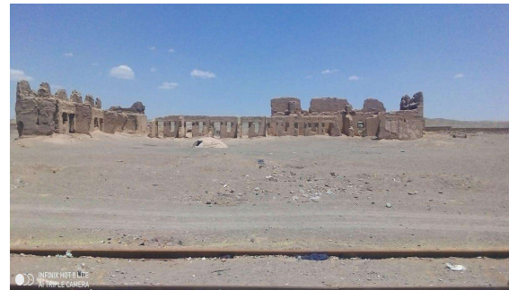
General view of old Taftan Railway Station from the south
