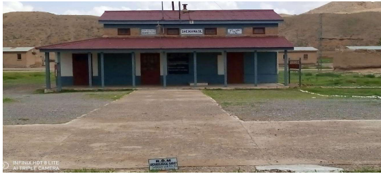
Façade elevation of Shaikh Wasil Railway Station from the east
