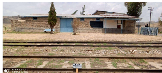
Northern façade elevation of Kishingi Railway Station
