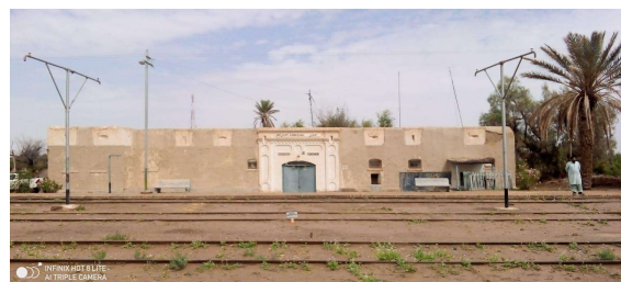
Eastern elevation of Ahmedwal Railway Station
