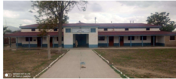
General view of Wali Khan Railway Station from the east
