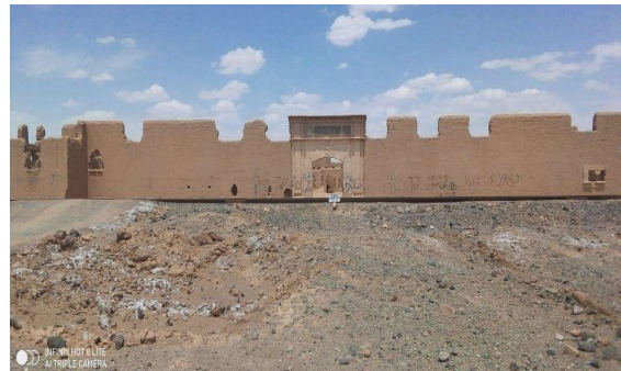
General view of Kundi Railway Station from the east
