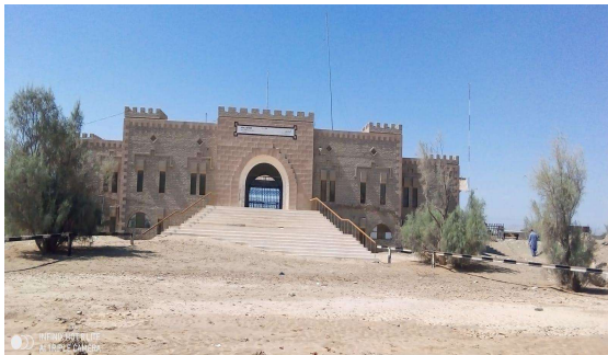
Façade elevation of Koh-i-Taftan Railway station
