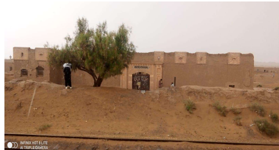
General view of Nok Chah Railway Station from the east
