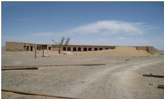
General view of Alam Raik Railway Station from the south
