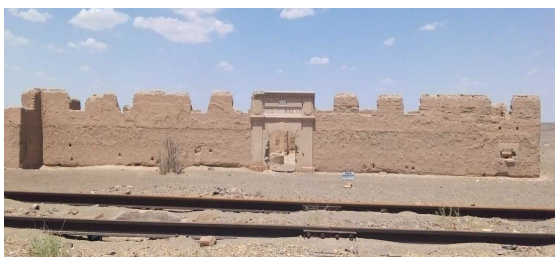
General view of Rag-i-Malik Railway Station from south
