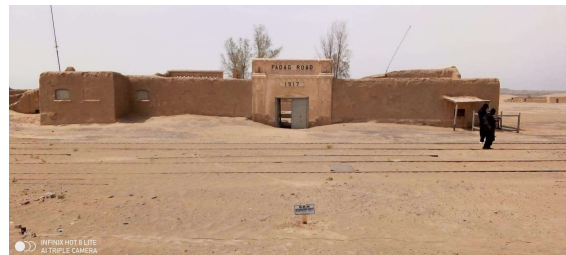
General view of Padag Railway Station from the north
