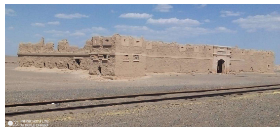
Southwestern view of Ware Chah Railway Station
