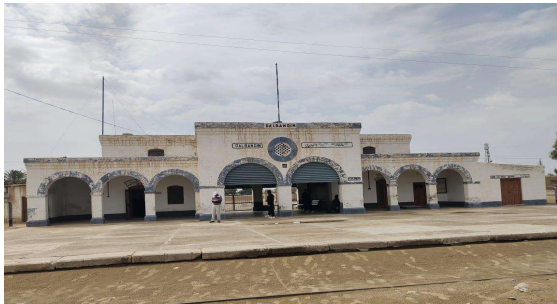
Inside view of Dalbandin Railway Station from the west
