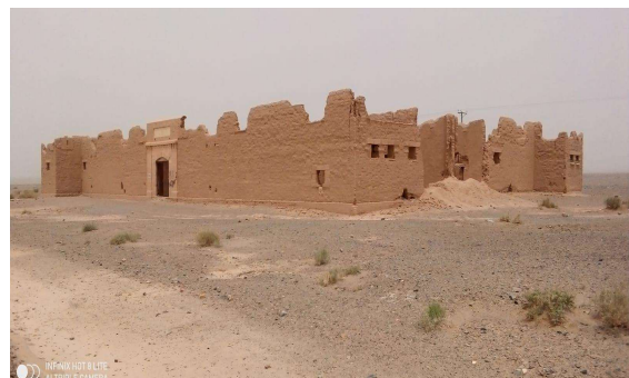
Northwestern view of ruins of Nuli Railway Station
