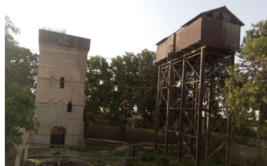
Water source at Kotri Settlement
