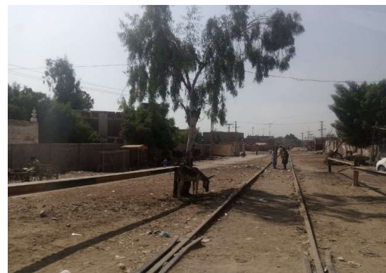
Railway Track near Dadu
