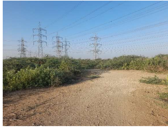
Un-sealed Road near Dhabeji Settlement
