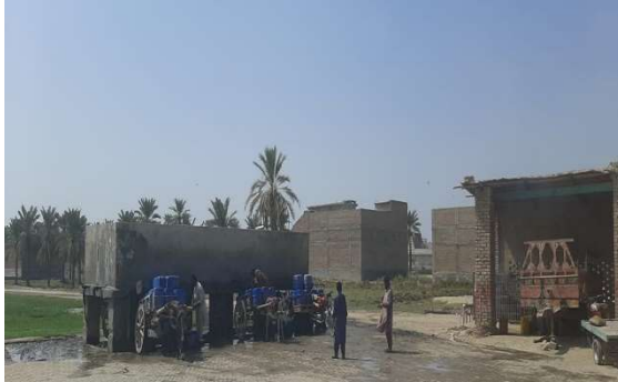
Water Filtration Plant at Jacobabad Settlement
