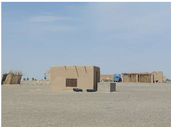
Kutcha House at Rajai Settlement
