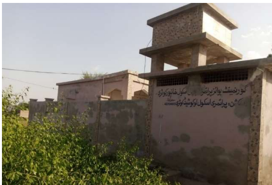
Government Boys Primary School at Kotri settlement
