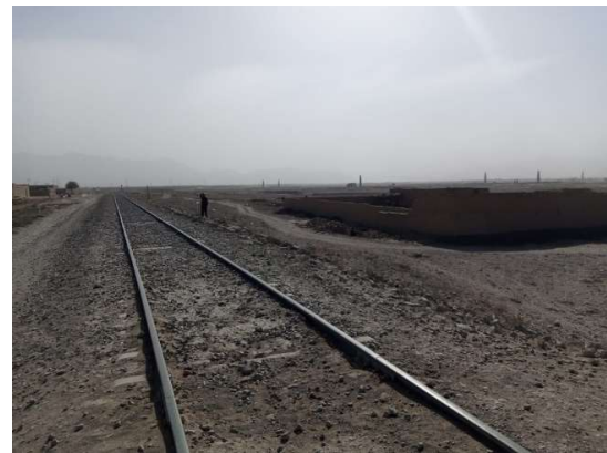
Railway Track near Spezand
