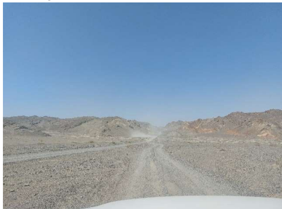
Un-sealed road near Kachau Settlement
