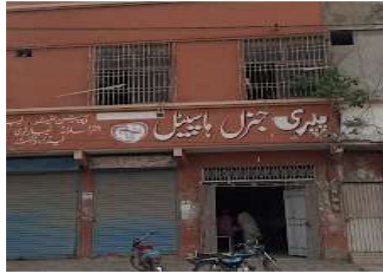
General Hospital in Pipri Settlement
