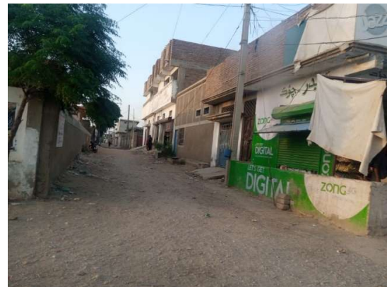
Un-sealed road at Larkana
