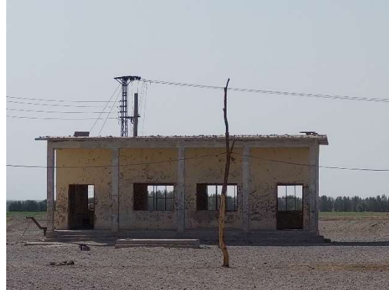
Primary School at Tahlab Settlement
