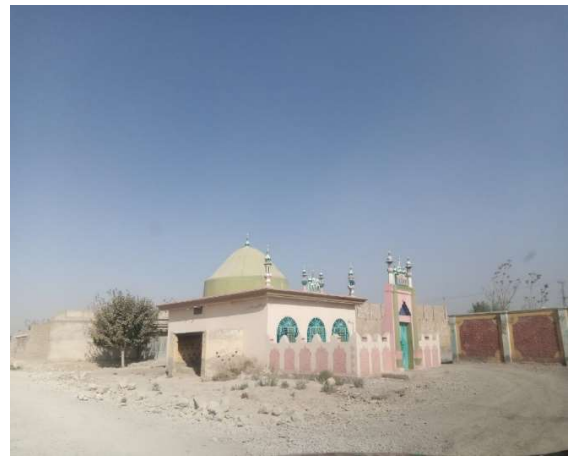
Mosque at Spezand settlement
