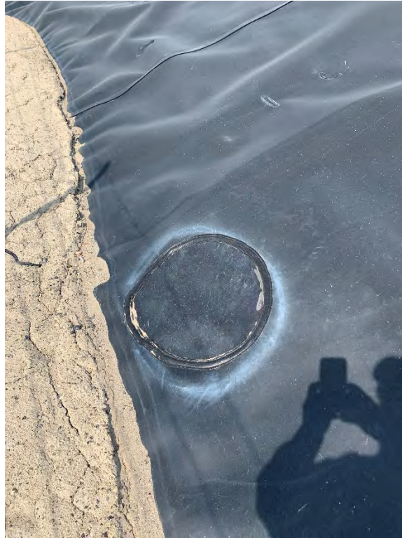
Photo 20. Liner Repair – Cell 1 South Bern Downstream Toe
