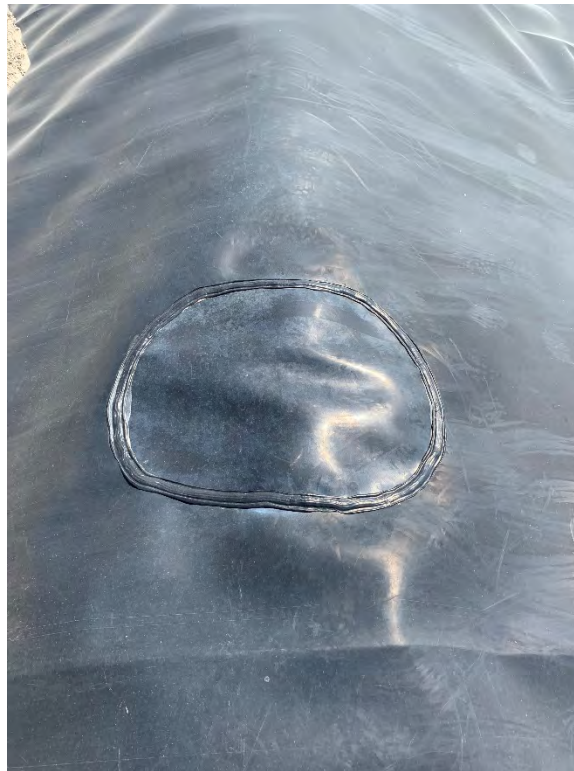
Photo 19. Liner Repair – Cell 1 South Berm Crest
