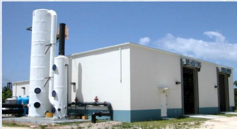
North Sound Plant – Grand Cayman
