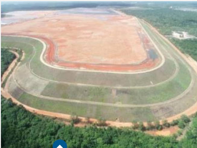
Alumar Residue Storage Area 5
