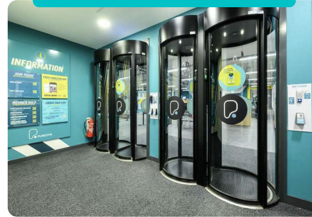
Automated access control
