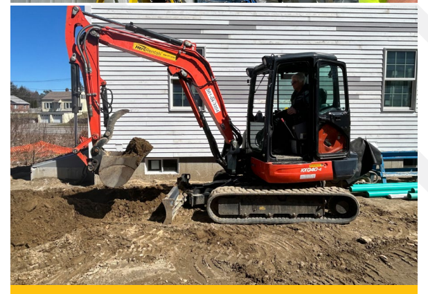
Donated excavator rental at Habitat affiliate's job site.
