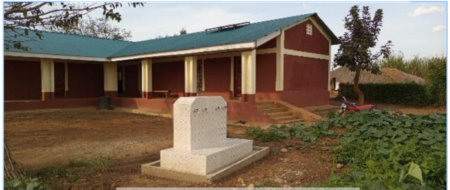
Renovation of the Renzi health centre
