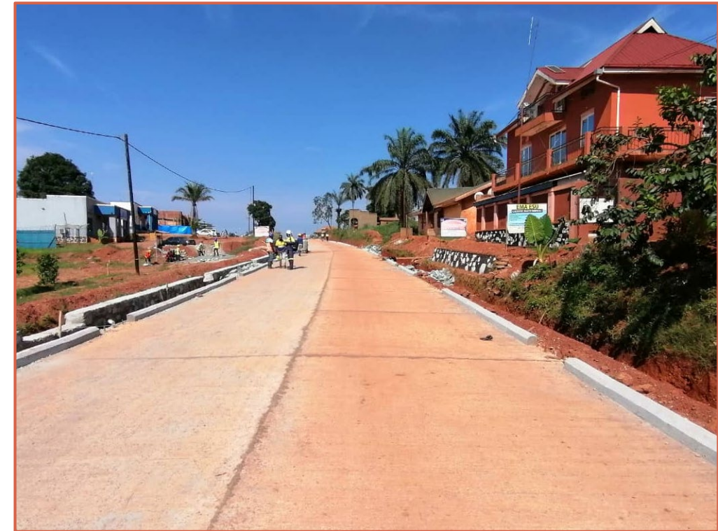
Construction of the asphalt road in Durba
