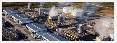
The Quisqueya 1 power plant began supplying power to the mine using natural gas in the first quarter of 2020. This conversion from fuel oil to natural gas is expected to reduce greenhouse gas emissions by 30% and nitrogen oxide by 85%, further reducing Pueblo Viejo's impact on the environment.
